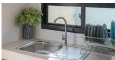
Kitchen Sink Fixing
