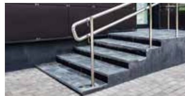
Staircases & Metal Railings
