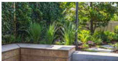
Fixing Stone on wall
